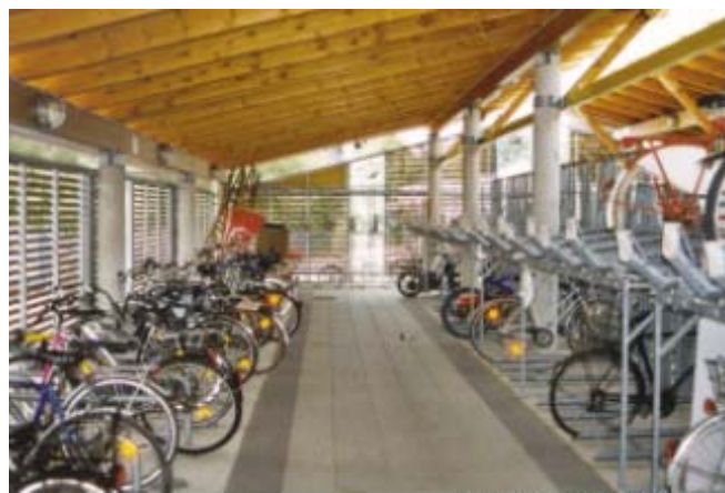
Cycle station, Bremen-Vegesack
